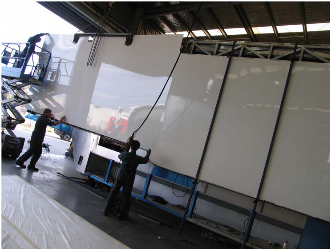
ABOVE: The panels being applied to the new ATA Mobile Education Unit.
